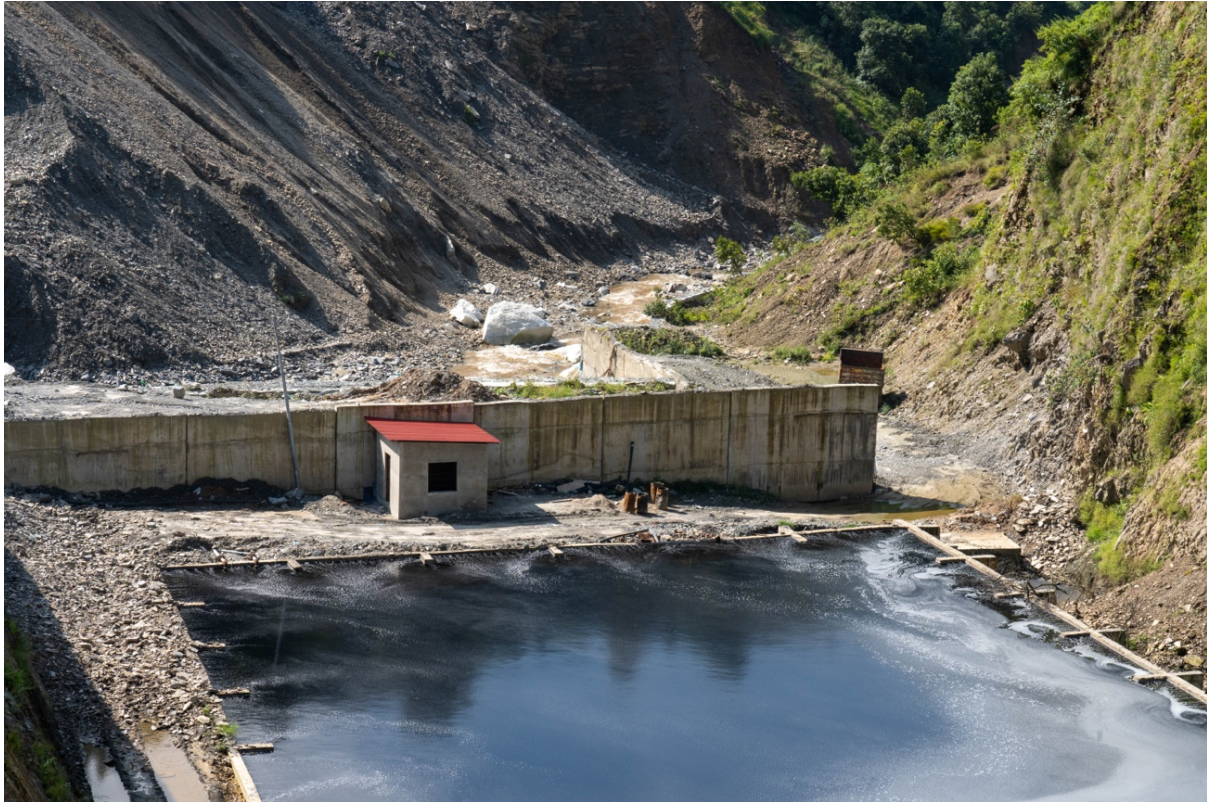
Figure 14: Overflowing leachate drainage system at Banchare Danda landfill
