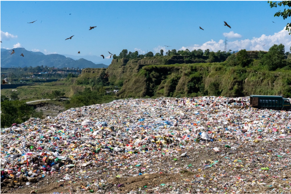
Figure 15: Overview of Pokhara landfill site
