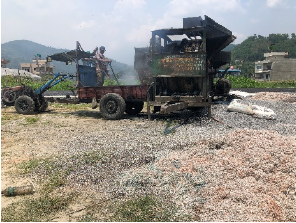
Figure 12: Plastic Road construction with manual method, June 2023
